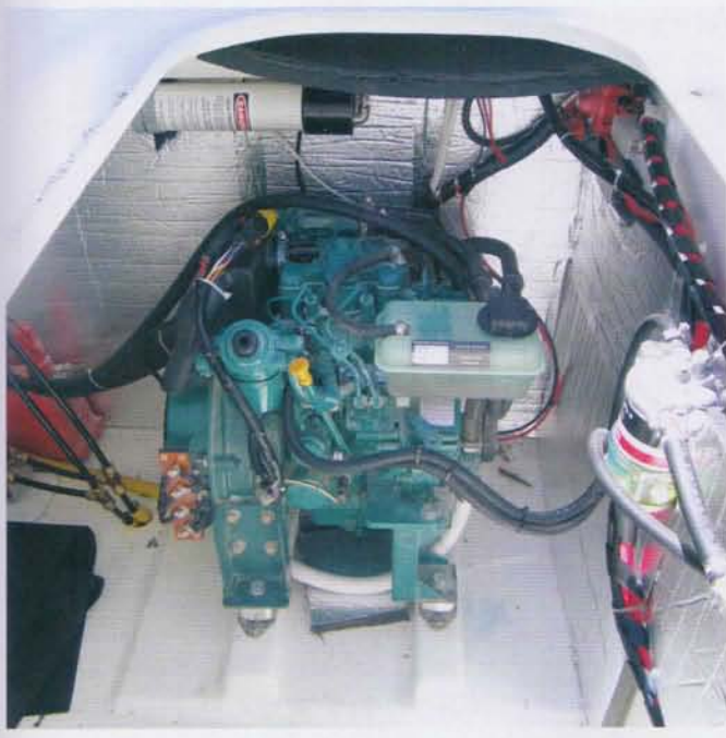
Volvo Penta 12.2hp diesel and 5.4kW 48 volt generator.
